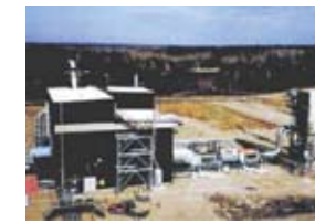
Staged Coal Combustor Plant for Steam Production
