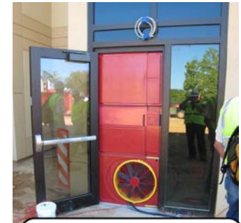
Air leakage test (blower door)
