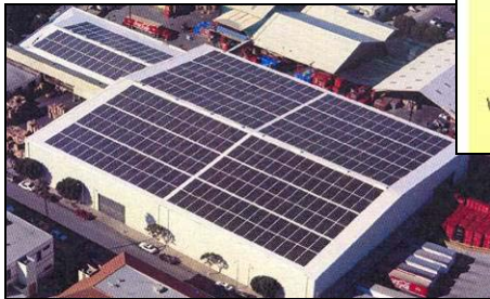
Renewable Power Production
